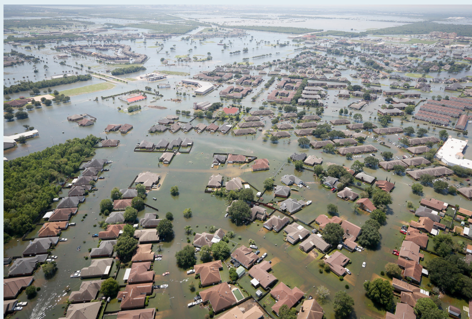
Figure 17.2: Hurricane Harvey led to widespread flooding and knocked out power to 300,000 customers in Texas in 2017, with cascading effects on critical infrastructure facilities such as hospitals, water and wastewater treatment plants, and refineries. The photo shows Port Arthur, Texas, on August 31, 2017—six days after Hurricane Harvey made landfall along the Gulf Coast. Photo credit: Staff Sgt. Daniel J. Martinez, U.S. Air National Guard.
